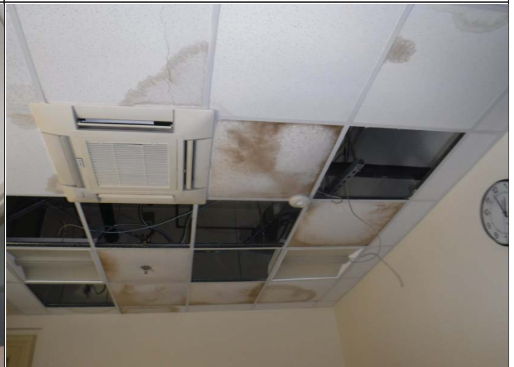
Caption #14: Damaged plaster ceilings – typical of 2 nd Floor Classrooms
