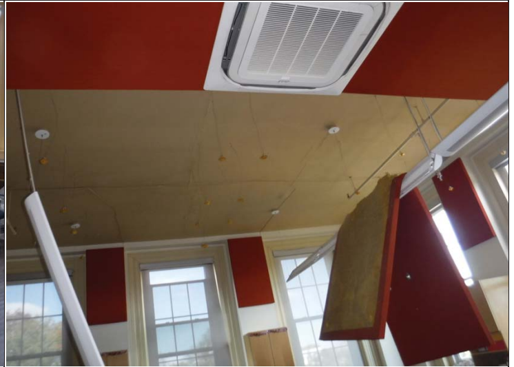
Caption #14: Damaged plaster ceilings – typical of 2 nd Floor Classrooms
