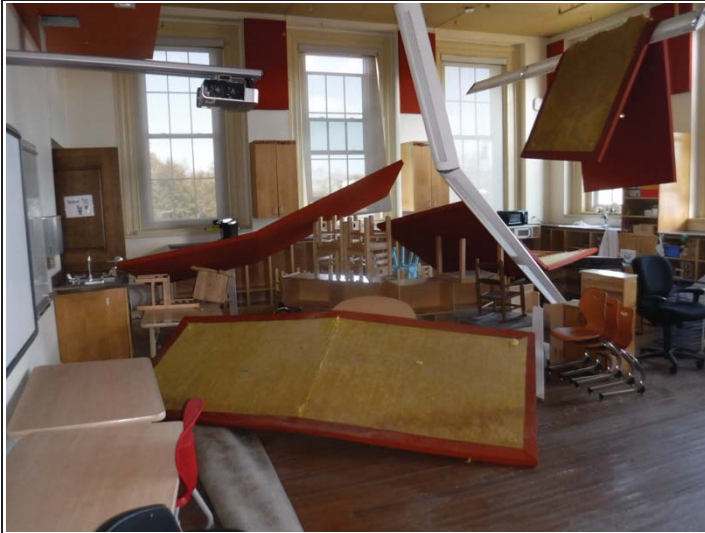
Caption #13: Classroom 203 damaged ceiling panels and lights – ( typical of 2 nd floor Classrooms)
