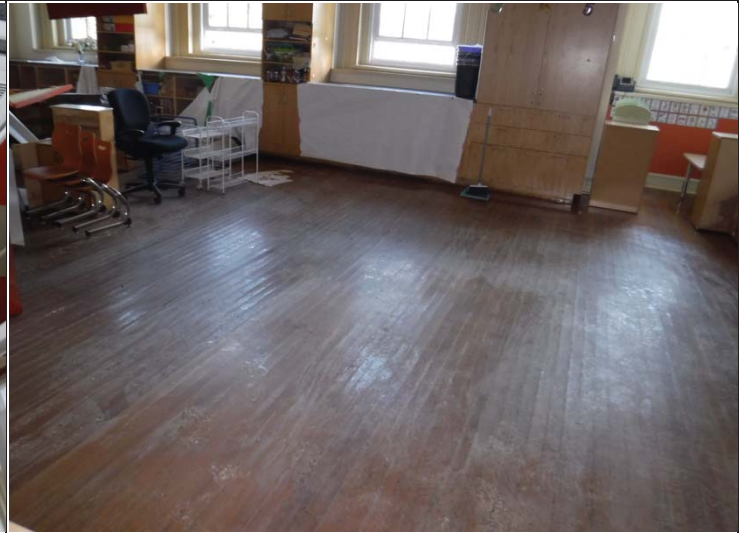
Caption #10: Classroom 203 condition at wood floors (typical at 2 nd Floor Classrooms)
