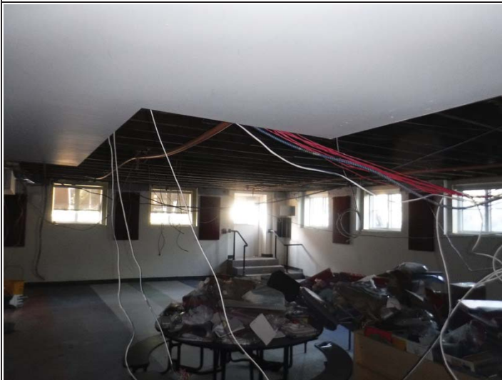
Caption #25: Kitchen 003 damaged ceiling and light fixtures
