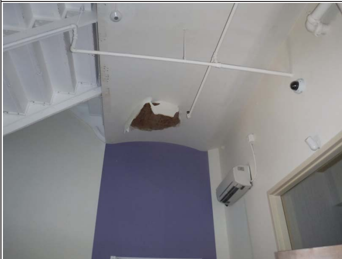
Caption #13: Classroom 203 damaged ceiling panels and lights – ( typical of 2 nd floor Classrooms)
