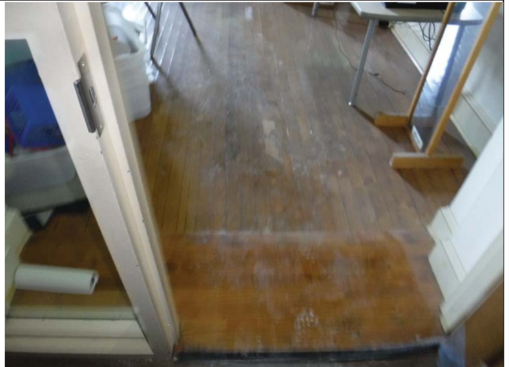
Caption #6: Floor condition at Classroom 307 and typical of wood floor condition at 3 rd Floor Classrooms
