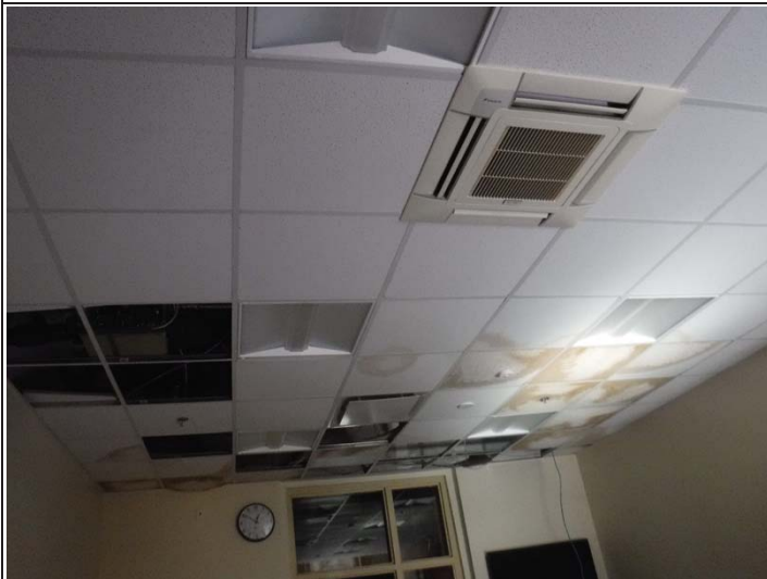
Caption #9: Classroom 206 damaged ceiling panels and light fixtures (typical at 2 nd Floor Classrooms)
