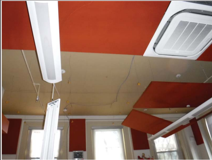
Caption #9: Classroom 206 damaged ceiling panels and light fixtures (typical at 2 nd Floor Classrooms)
