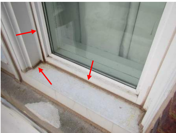
Photo 11: Sill of new window at auditorium. Arrows highlight field installed sealants at metal-to-metal joints/seams.
