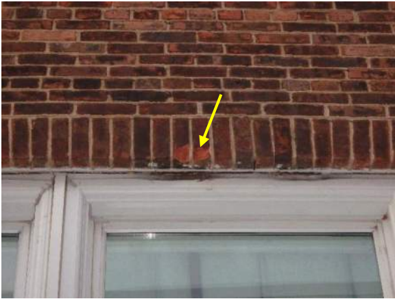
Photo 7: Brick spall above window.
