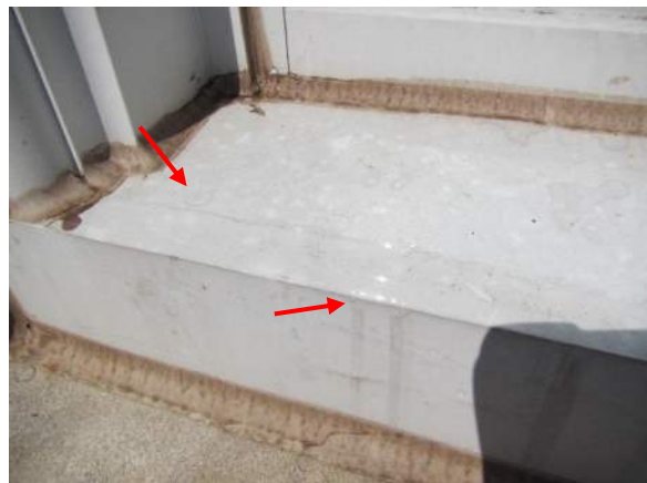
Photo 12: Close-up view of sill/jamb interface. Arrows denote water on sill framing.
