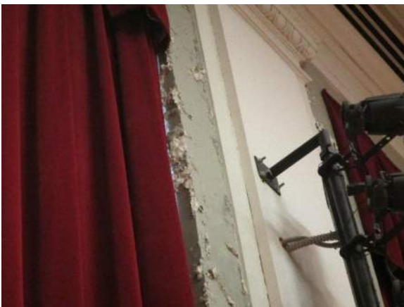
Photo 17: Deterioration of plaster at window jamb.
