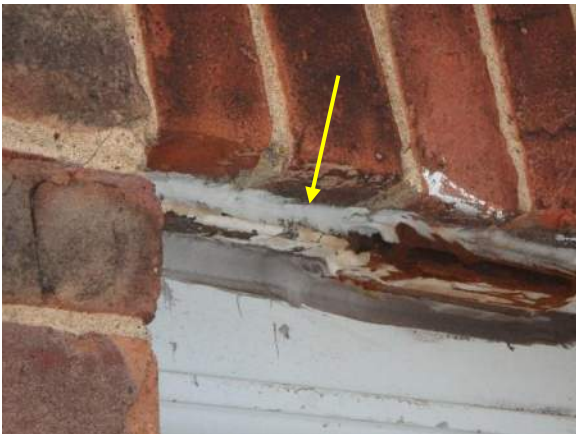
Photo 9: Sealant installed between soldier brick and steel lintel.
