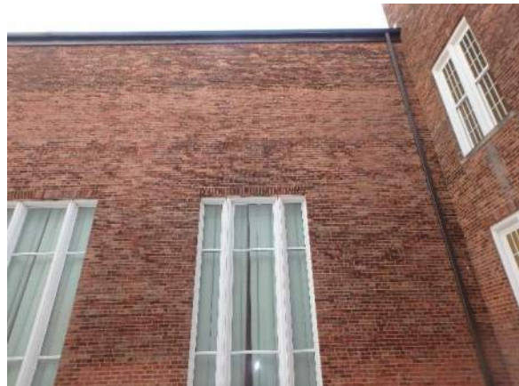
Photo 10: Partial view of west exterior wall of auditorium. Note varying color and staining of brick.
