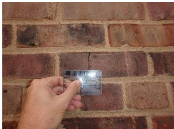
Photo 6: Crack through brick.
