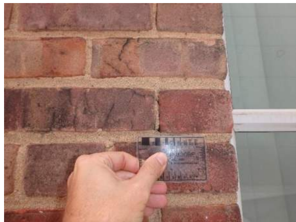
Photo 4: Mortar joint void.
