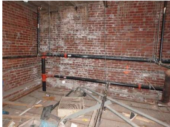
Photo 20: Efflorescence observed inside attic.
