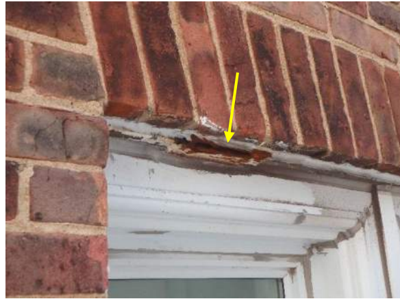
Photo 8: Corrosion at window head.
