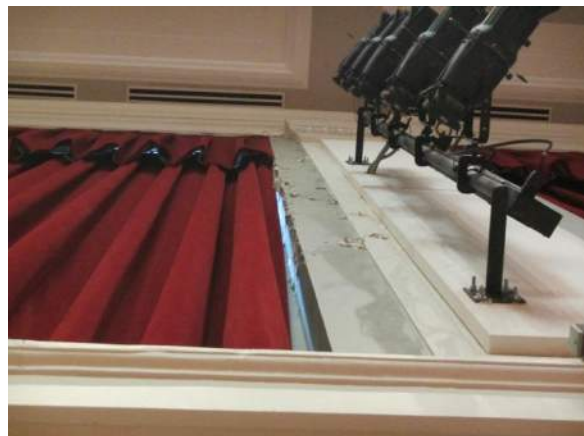
Photo 18: Deterioration of plaster at window jamb.
