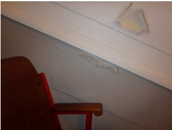
Photo 15: Peeling paint at east wall at balcony.
