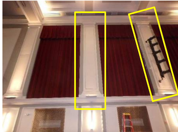
Photo 14: Closer view of windows on west wall. Areas of most prominent moisture-related distress are highlighted.
