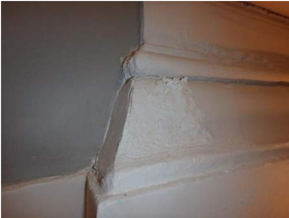
Photo 19: Deterioration of decorative gypsum shape near window sill.
