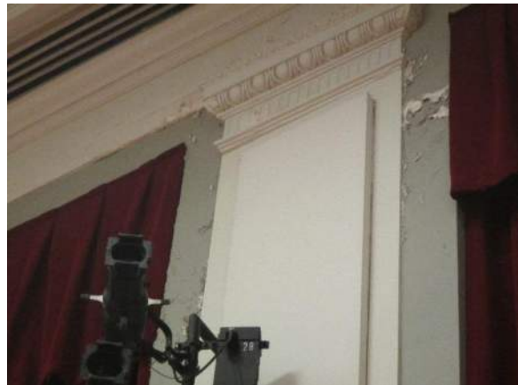
Photo 16: Plaster deterioration between windows.
